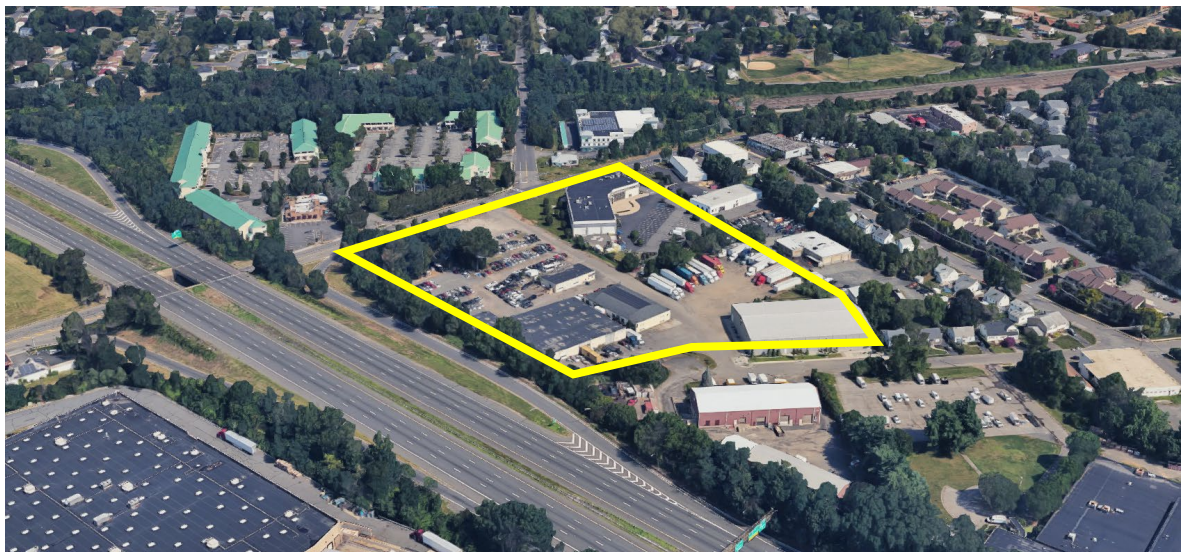
Screen Capture from Google Maps looking north; Property outlined in yellow, fronting Middlesex Avenue (top) and High Street (bottom).
