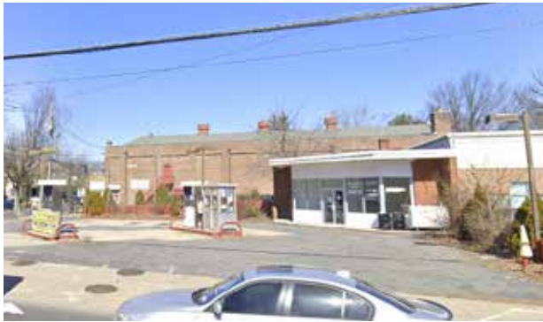
Vacant gas station, looking north
