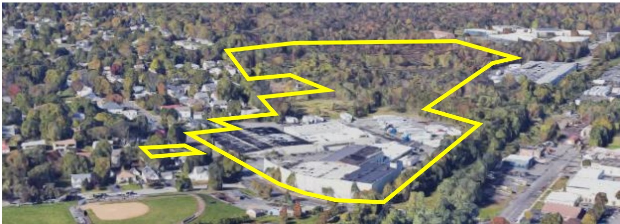
Bird's eye view of the Project Area, looking northwest, outlined in yellow. Source: Google Maps; screen capture on September 9, 2021. The Project Area is generally bounded by Durham Avenue (bottom and to the left), the future Middlesex Greenway Extension (right) and Peter J. Barnes III Wildlife Preserve (top).
