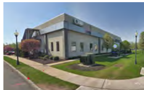
Cross County Powersports, facing south.
