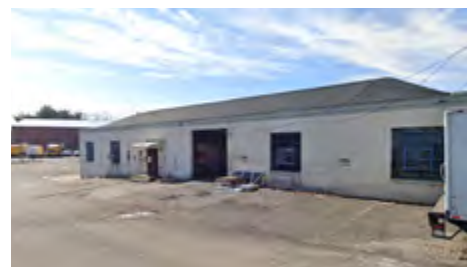
Light Industrial building, facing west.
