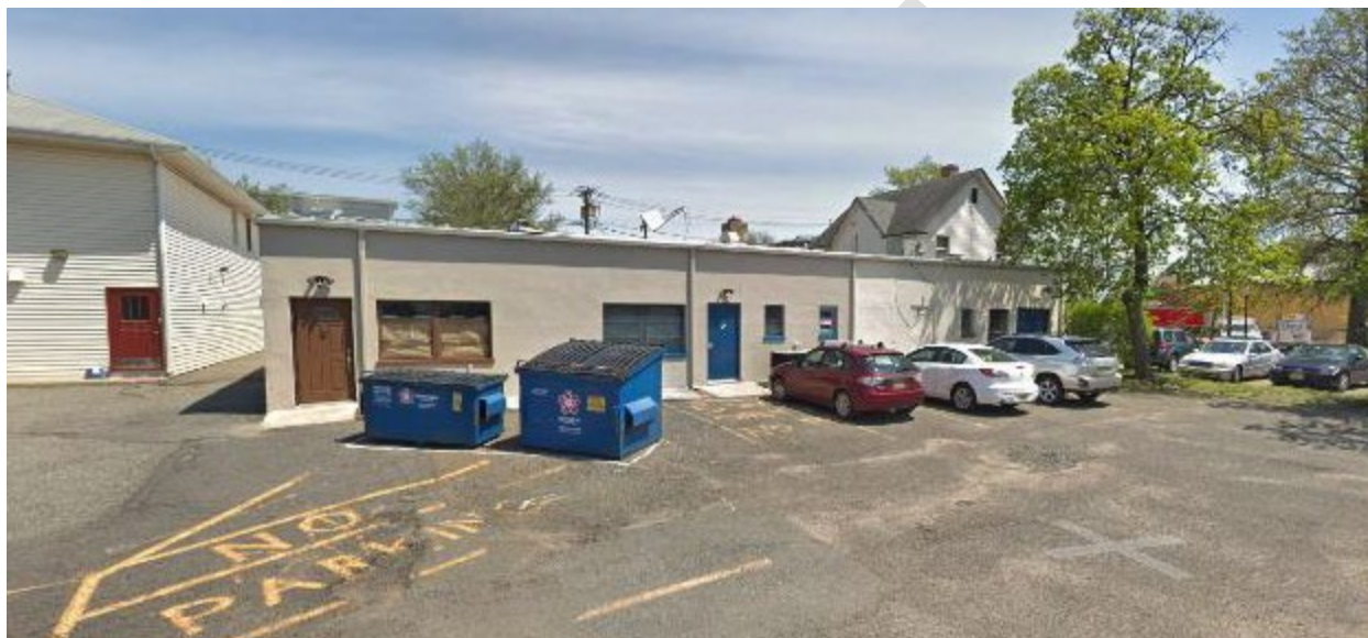
Figure 9. Google Street View of rear parking area, which has since been repaved.
