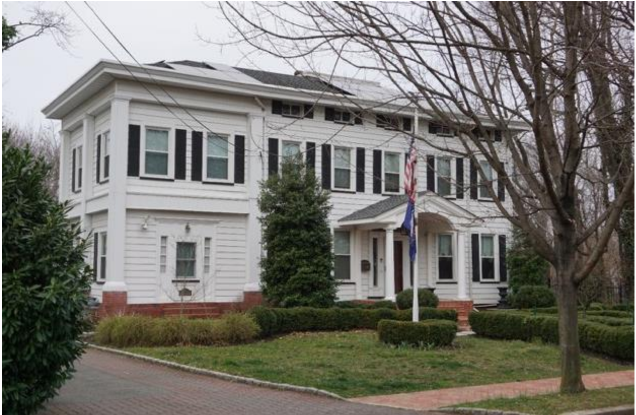
Photograph 12. Governor Silzer's House at 79 Graham Avenue
