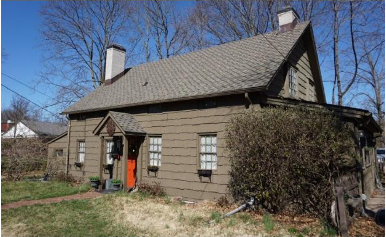
Photograph 9. Ayers-Allen House at 16 Durham Avenue
